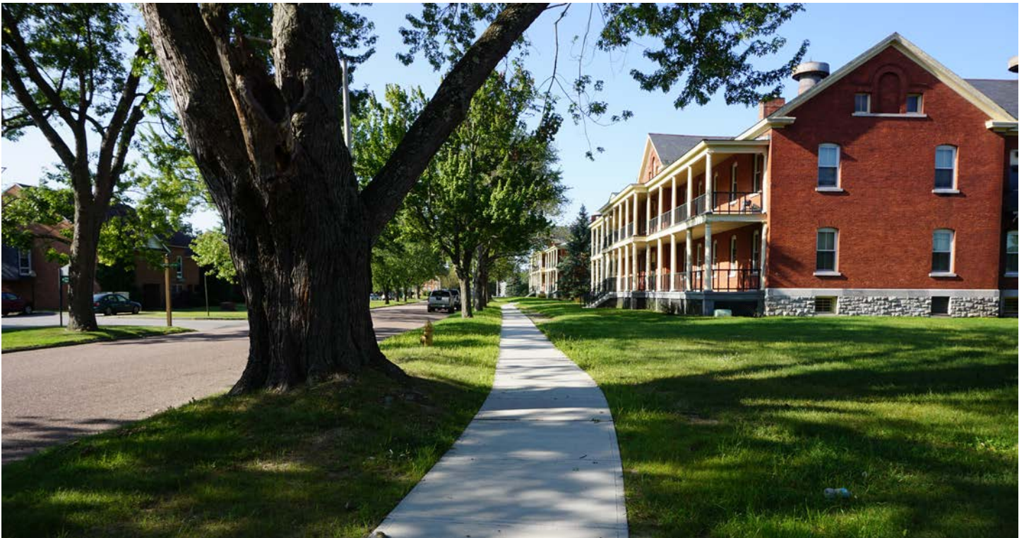
Fort Ethan Allen Sidewalk, Colchester, Vermont
